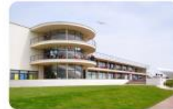
De La Warr Pavilion, England
